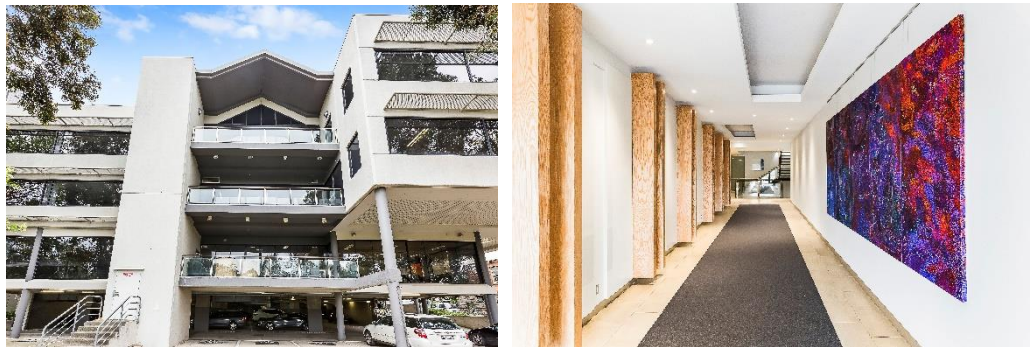
Images L to R, top to bottom: façade of 675 Victoria Road, Abbotsford, exterior of property including carpark, internal corridor on site.
