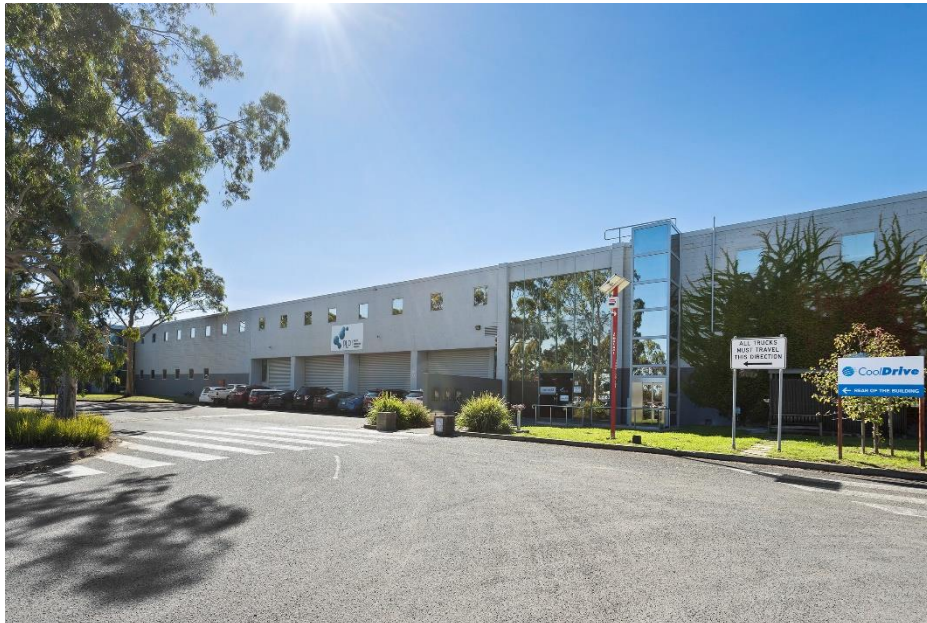
Below: 15-33 Alfred Street, Blackburn.
