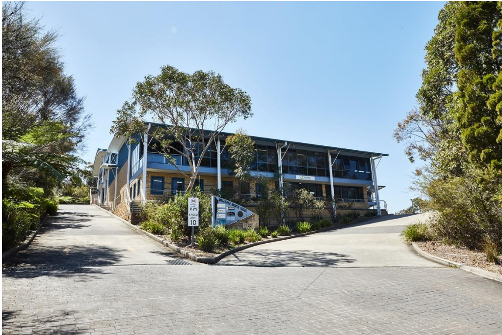
The façade of 22 Narabang Way, Belrose.
